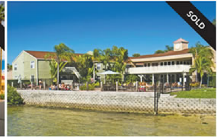
Prestigious Multi-Family Complex | 205 CAs Signed 689 Units | Tampa, FL | 95% Leased
