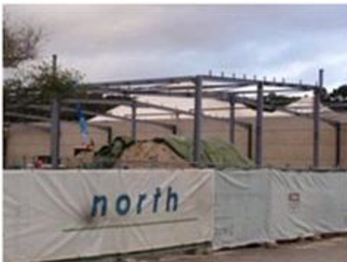
Casey's Toys rebuild well underway.
