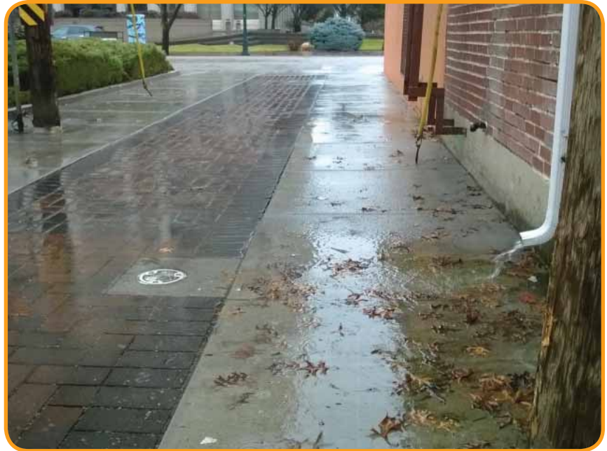
Permeable paver alley
