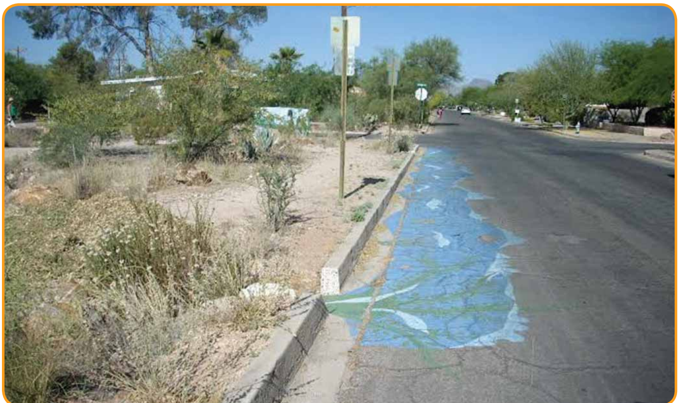
Painted curb cut
