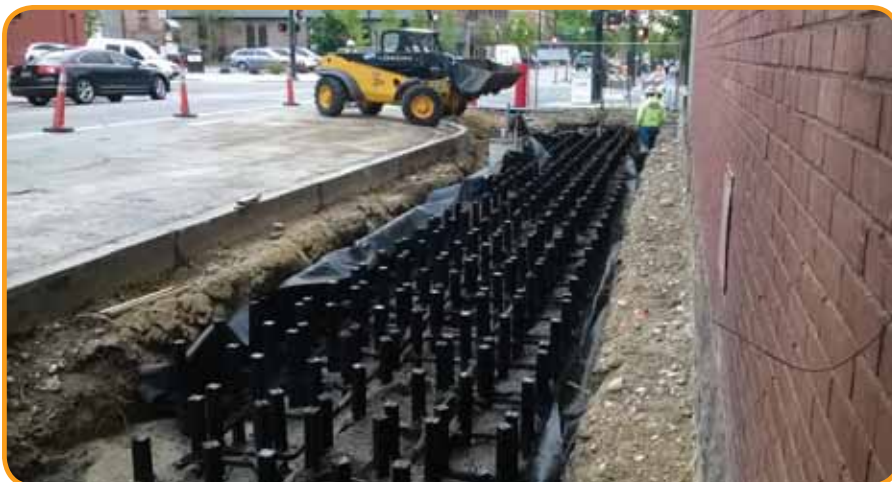
Silva Cell installation
