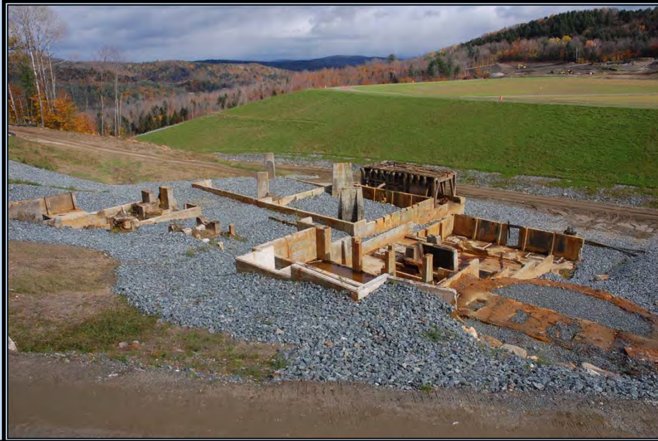
WWII Building Foundations from Site Access Road
