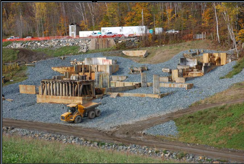
WWII Building Foundations from TP-1
