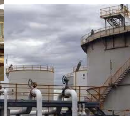
Department of the Air Force, HQ 72nd Air Base Wing (AFMC), Tinker Air Force Base, Repair/Replace Industrial Waste Treatment Plant (IWTP). Oklahoma City, OK.
