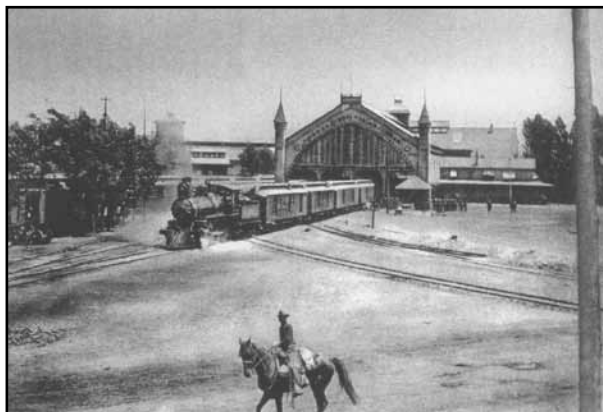
Central Pacific Railroad Depot, 1897
