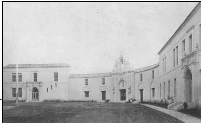
The just completed school at 21st Street, 1925
