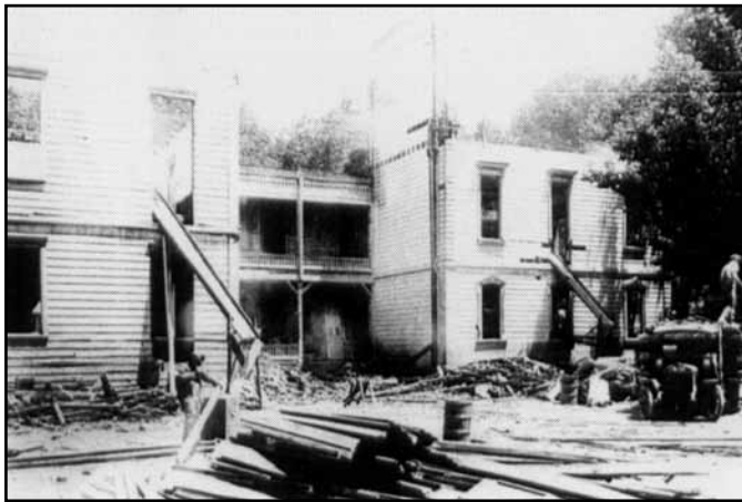
The dismantling of the original Christian Brothers College, 1923.
