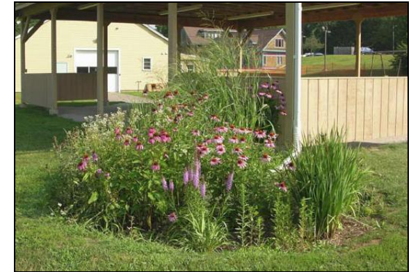
This rain garden in Vernon, CT was constructed as a demonstration project to treat and infiltrate runoff from an outdoor pavilion. Photo: USDA NRCS
