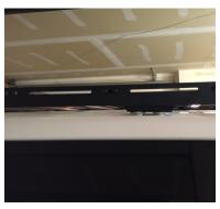
In some cases due to minor changes in the roof lines extra fender washers may be needed to level the rack at the mounting points.
