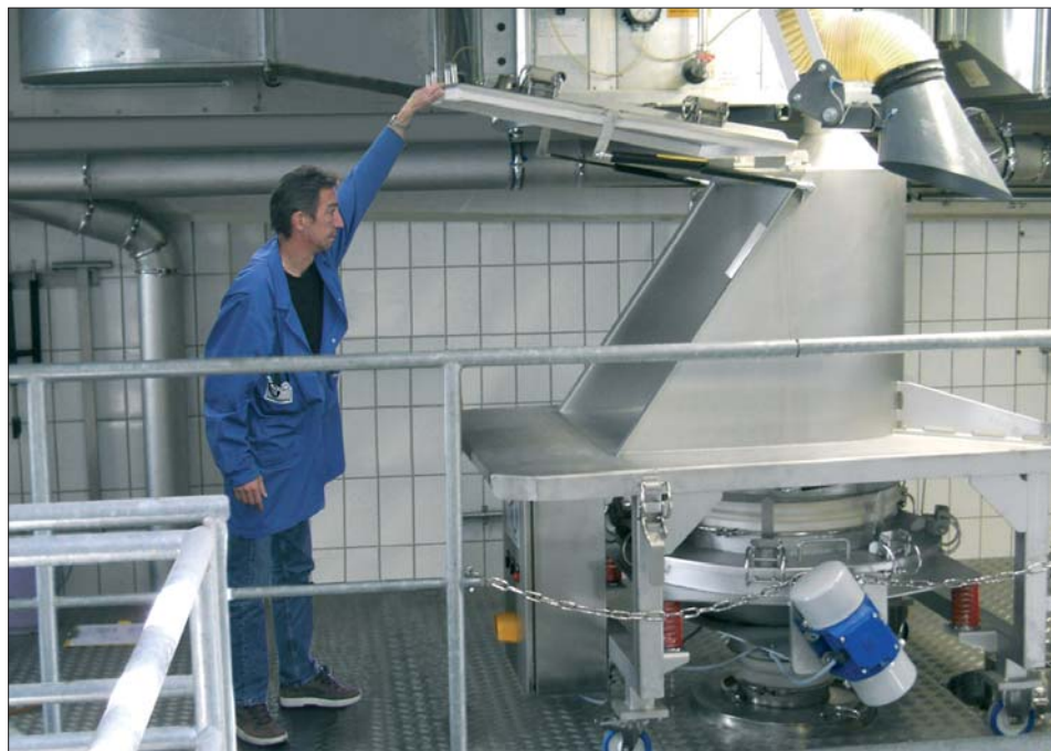
Round screening machine in a bag tipping station
