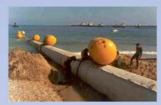
The Minor Totally Enclosed liftbags range from 50Kg (T1C) to 500Kg (T10C) lift capacity, with a safe working load of 6:1. Each bag has heavy duty webbing straps, anchor points, shackles, inlet/outlet valve and over pressure relief valve.
