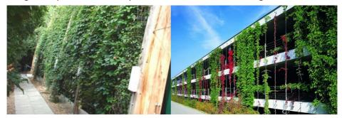
To aid the climbing process on buildings a number of systems exist including wire mesh frames, trellises and steel cables. The use of each frame is guided by the individual application, for example ivy plants grow easily and can attach themselves to walls and the side of building with minimal additional intervention. Often frames will be used to encourage the direction of growth or to support different species of plant growing on the wall.
