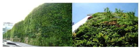
The natural water retention properties of most substrates allow irrigation systems to be simple in design and construction, thus lowering installation and maintenance costs. However, an associated disadvantage of substrate-based systems is their weight relative to other solutions. Newer lightweight materials are increasingly becoming available to address this issue.
