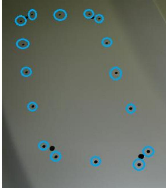
14) Use the stepped bit to enlarge the corners of the area you will be cutting out to ¼ inch or larger.
