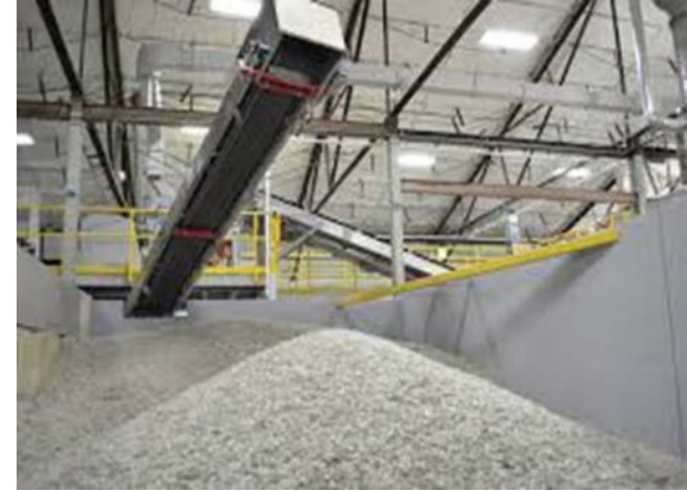
Flint glass storage area- Rumpke Glass Plant- Dayton, Ohio
