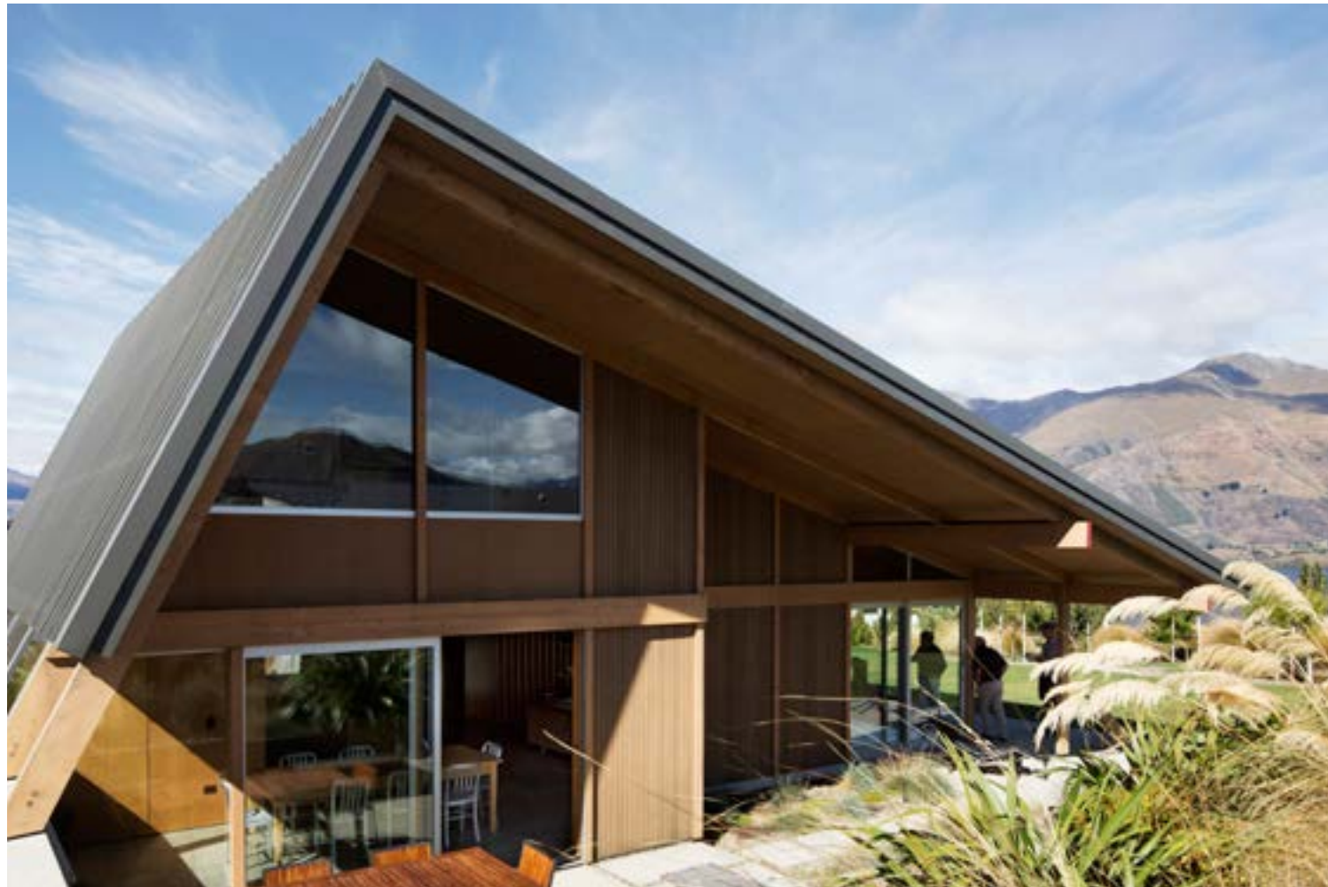
Above Low, west-facing eaves ensure the house never overheats in summer, yet enable the concrete floor to collect and distribute heat in winter.
