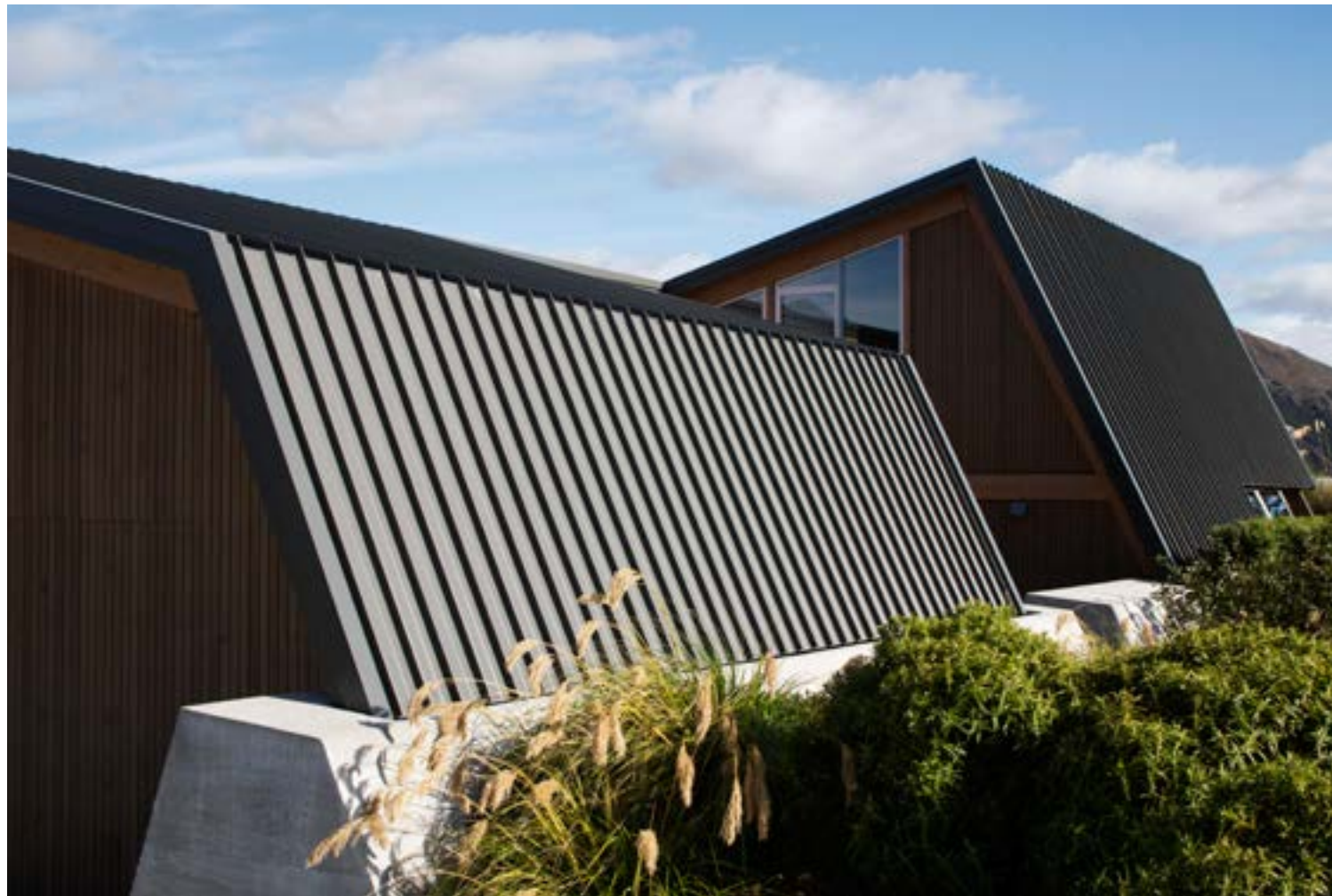
Above By cutting into the site and lowering the building platform by about a metre, the home is able to snugly hunker down.
