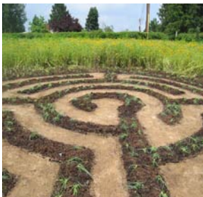
Installation of Labyrinth
