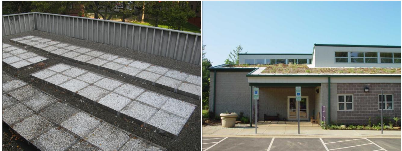
Figure 4: A blue roof consisting of engineered trays with stone ballast (left) and a green roof tray system installed on a sloped roof (right)
