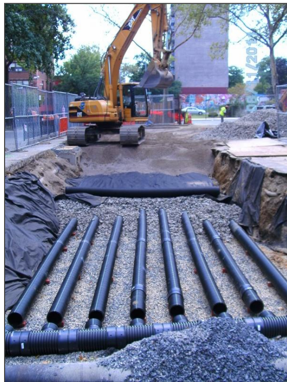
Figure 3: Subsurface chamber (top) and perforated pipe (bottom) infiltration systems under construction
