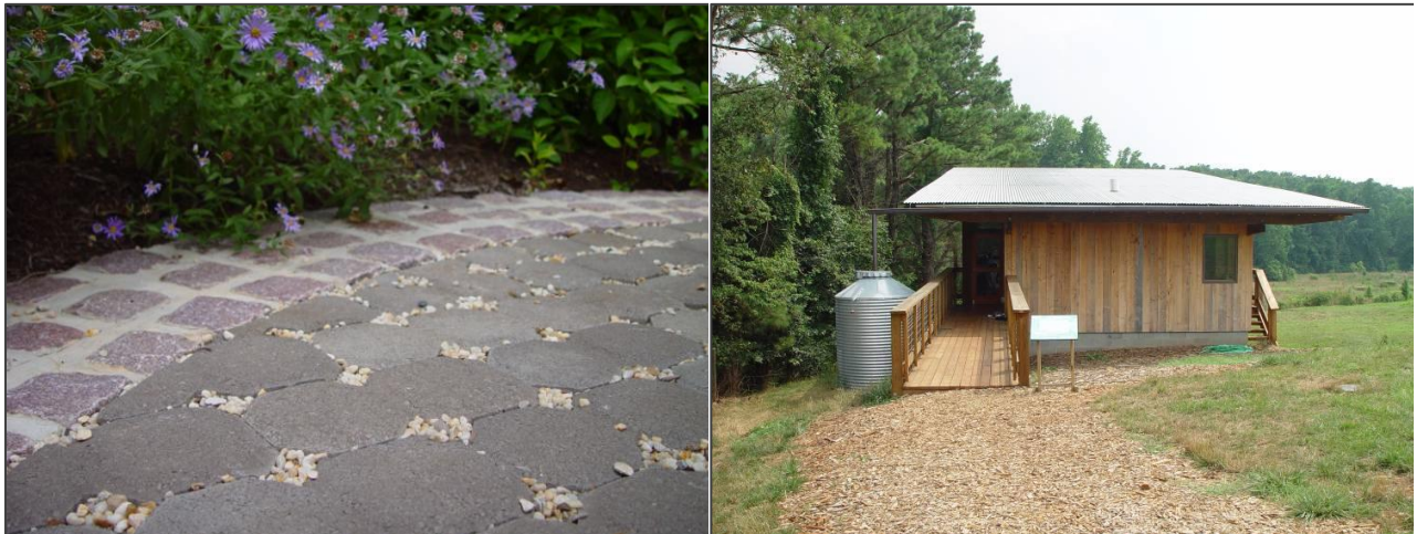
Figure 5: Perimeter of a permeable pavement walkway (left) and a rainwater harvesting system installed at a nature education center (right)
