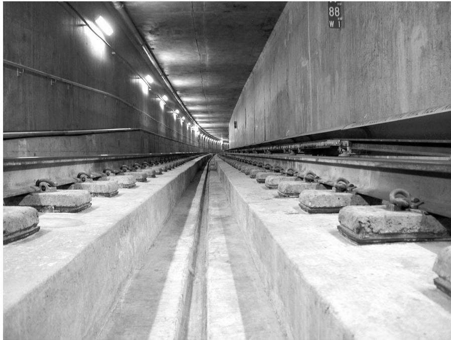
Fig. 7. Photograph of resiliently supported half ties (LVT track) in the San Francisco Airport Extension subway.
