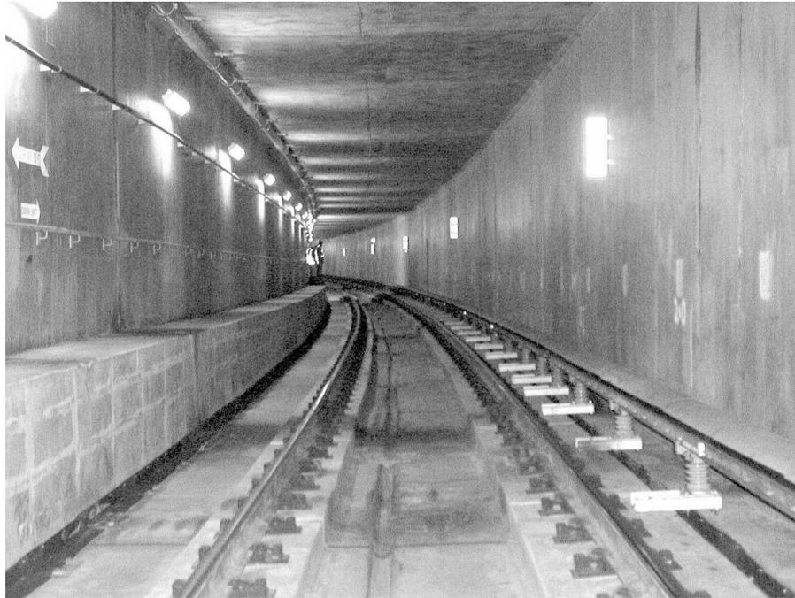
Fig. 8. Photograph of continuous floating slab track section in the San Francisco Airport Extension subway. Because there are no gaps between the floating slab and the subway invert larger than a few inches, impact testing from the invert to the surface was not feasible for this section of track.
