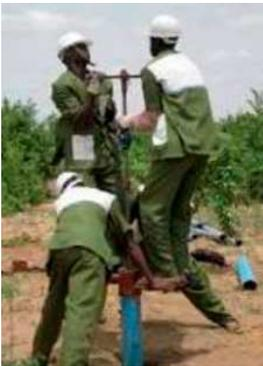
They've drilled those small diameter holes to an average depth of 18 m. And cased them with some perforated casings.
