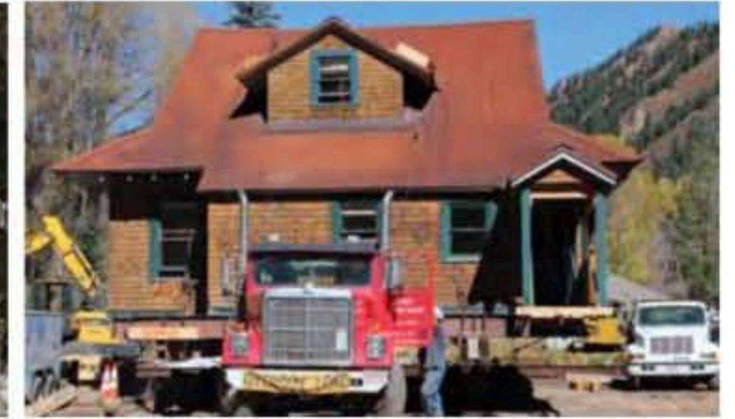
Left: A view over Castle Creek of the buildings in mid-build this past winter. Right: The 1890s Newman Bungalow, the home of the foreman of the Newman Silver Mine that occupied this site at that time, was picked up and moved about 150 feet to allow for better site design.
