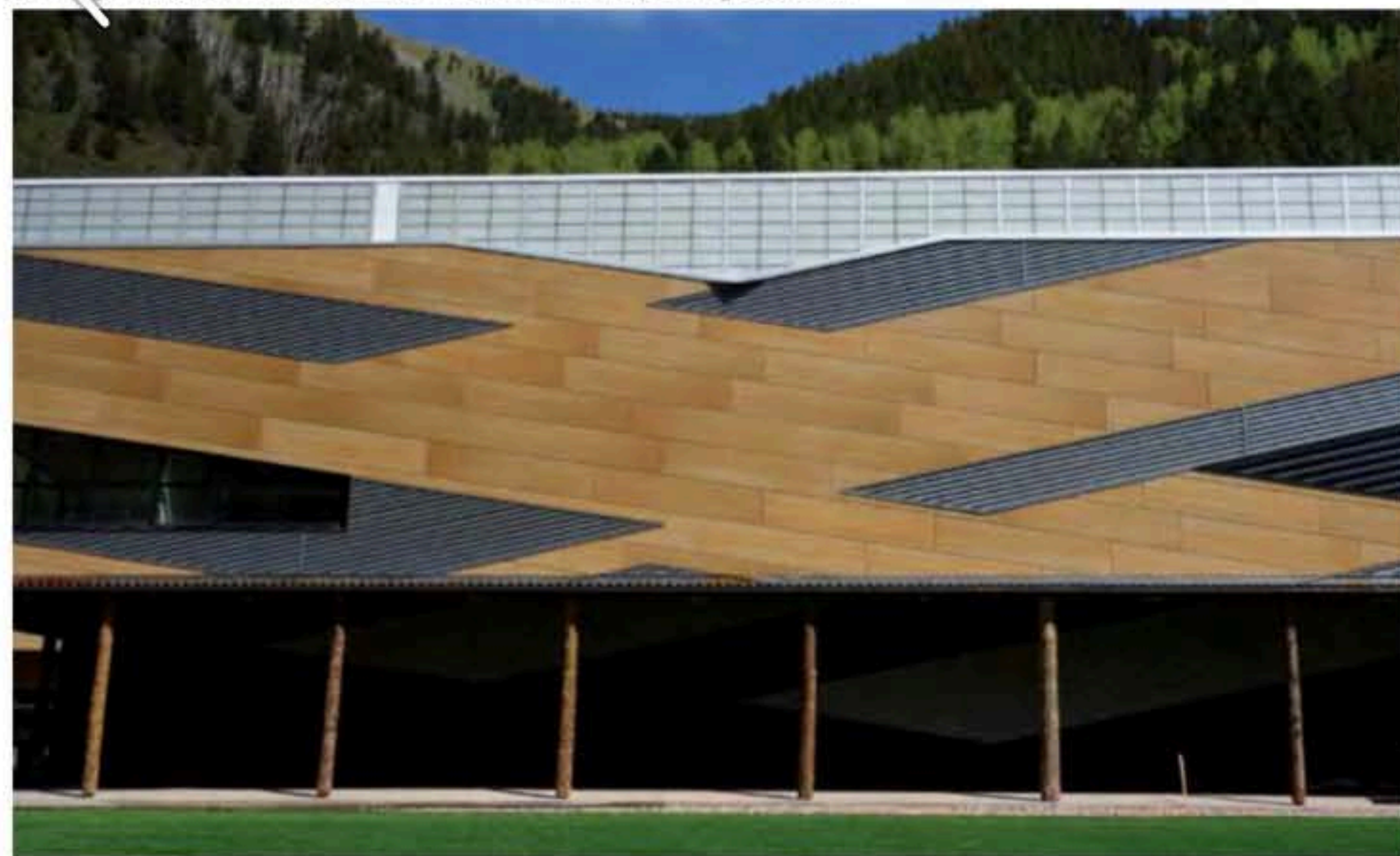
A large romantic orchestra can rehearse in the 7,400-square-foot Hurst Hall. The building has extra light for acoustic "bloom" to mimic the sound blend and carry of a large auditorium.
