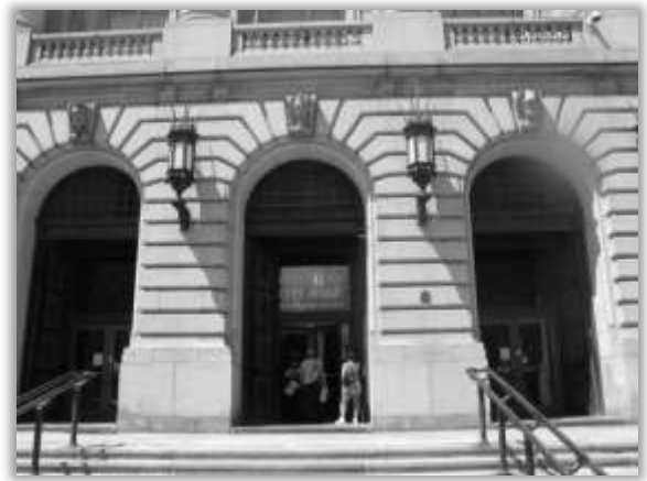
Cleveland City Hall
