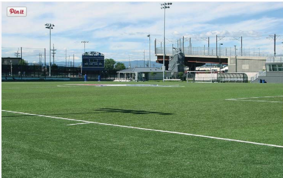
Completed soccer fields
