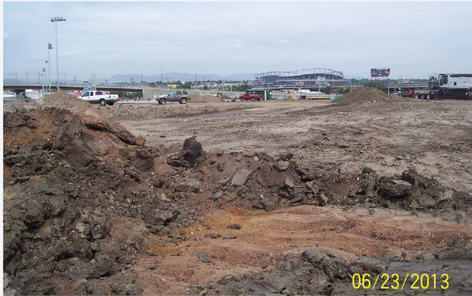
Brownfield site at start of construction
