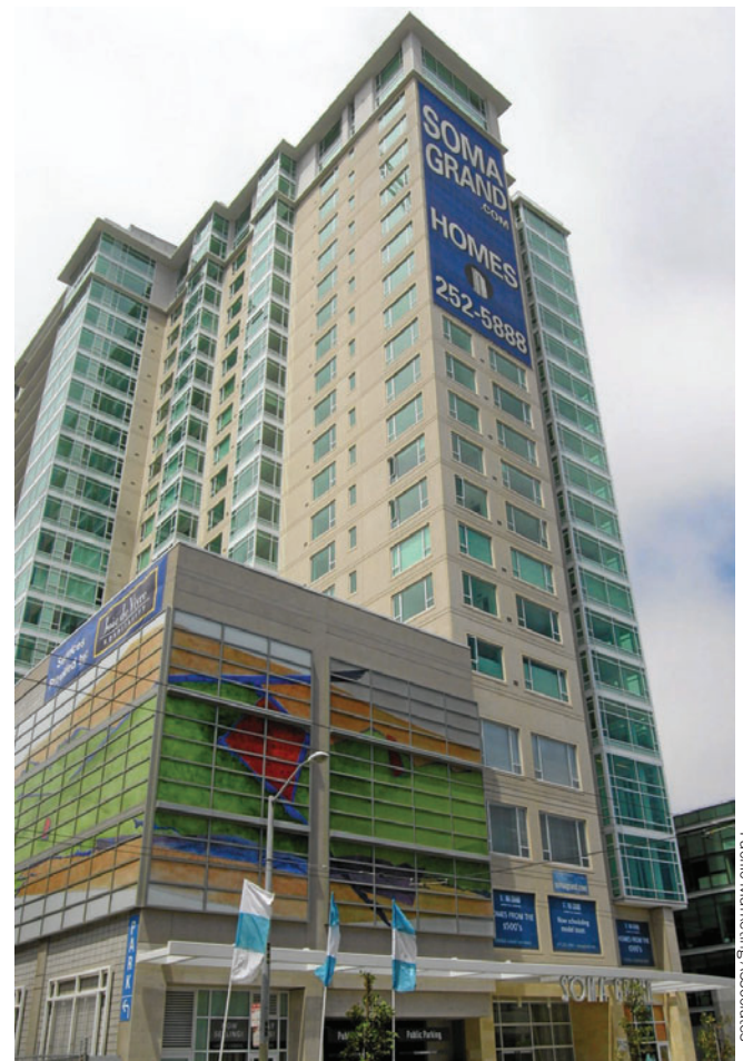
SOMA Grand was built in 2007 with 246 luxury condominiums. Located in San Francisco, it includes 29 below-market-rate units sold to households earning at or below median income.
