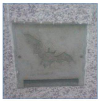
Permanent bat boxes installed in external wall insulation to counter the detrimental effect construction could have on bat populations.
