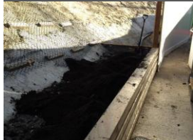
Step 2 Building the planter
