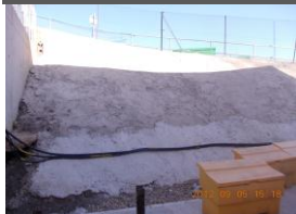
Step 1 Concrete batter
