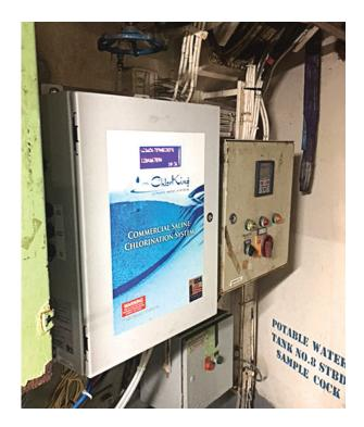
Compact ChlorKing Chlor SM salt chlorination systems for ships require minimal space. Maximum size for the power supply, shown here, is 20 in x 20 in.
