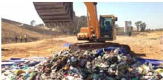
Operator needs to be under careful supervision to avoid the tarpaulin being pierced by the teeth of the bucket of the excavator
