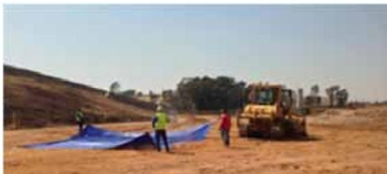
10m<sup>2</sup> tarpaulin is arranged to be ready to accept the waste load.
