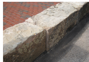
Recycled Bridge Abutment Benches at Greenfield
