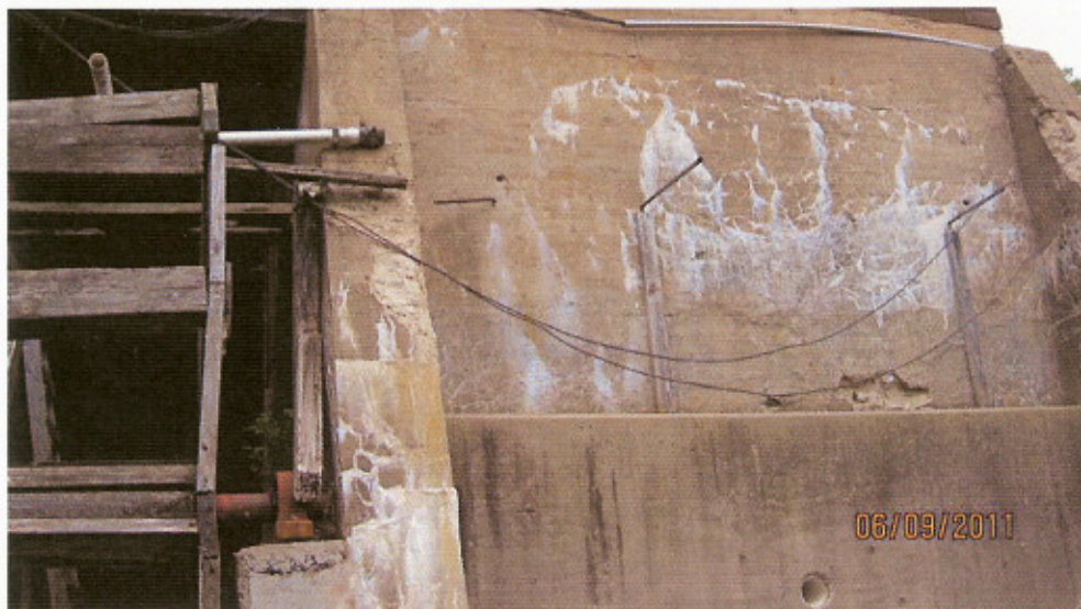
Rear Powerhouse Foundation Wall (0009300609201127)
