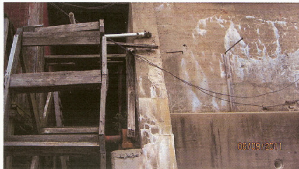
Rear Powerhouse Foundation Wall (0009300609201130)
