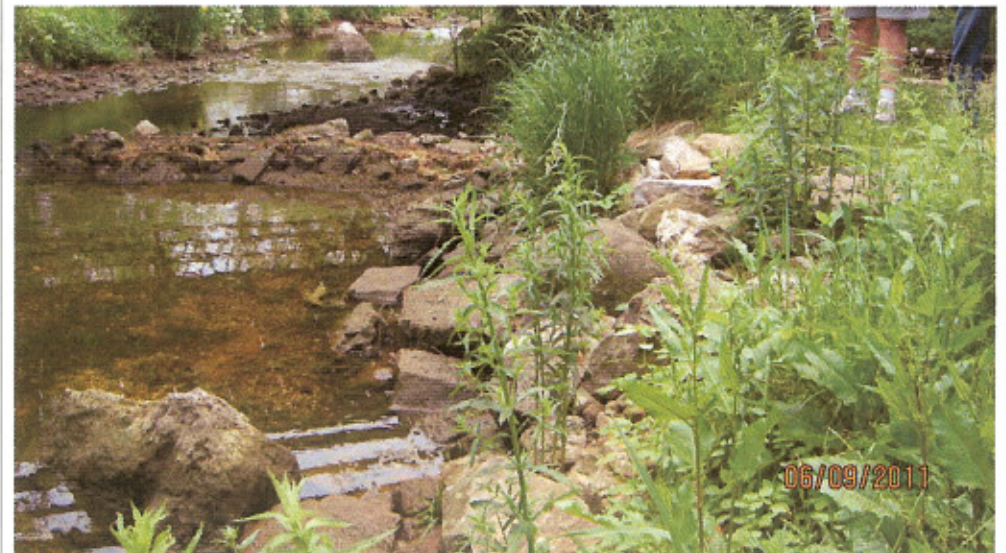
D/S Tailwater Channel Right Side (0009300609201135)
