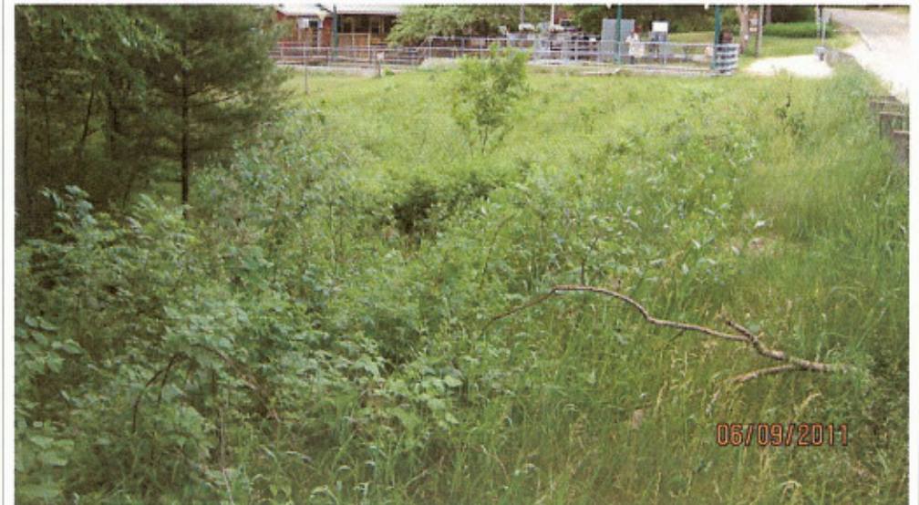
Left Side D/S Embankment - South (0009300609201112)
