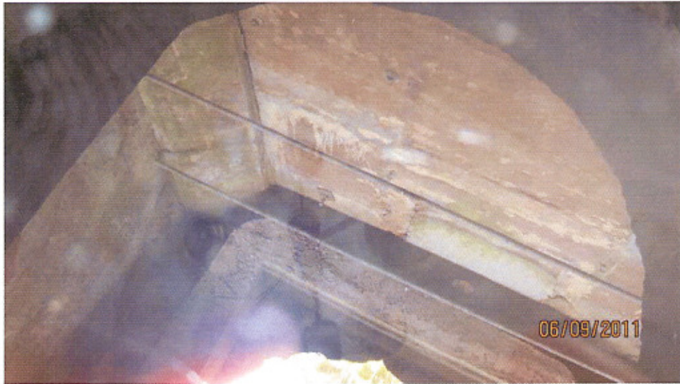
Powerhouse Head Race Rear Foundation Wall (0009300609201157)
