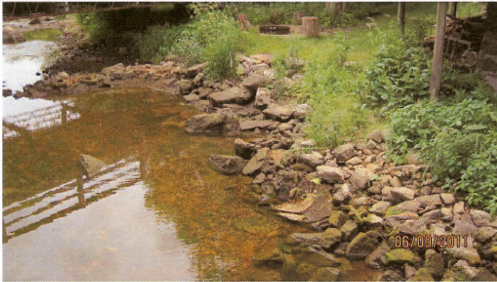
D/S Right Side Rip Rap (0009300609201151)
