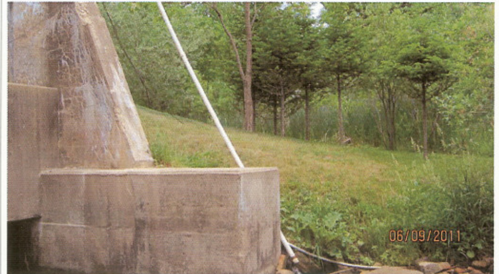
D/S Left Side Abutment / Bulkhead (009300609201122)
