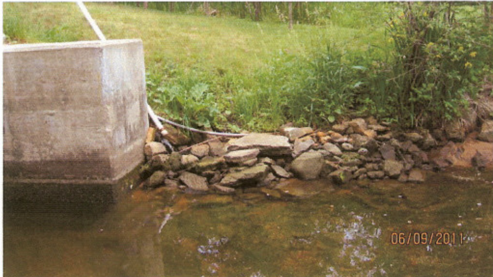
D/S Left Side Abutment / Rip Rap (0009300609201123)
