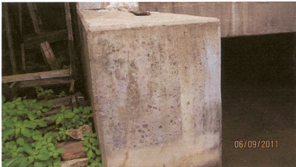
D/S Right Abutment (0009300609201125)
