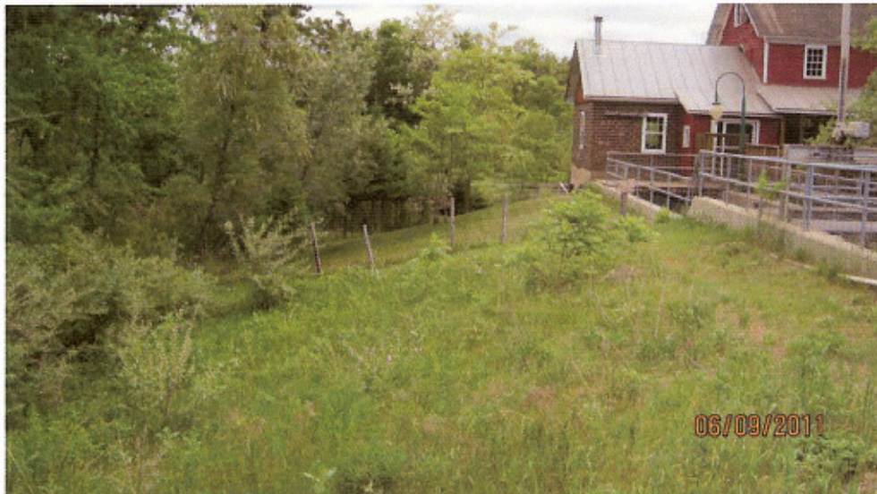
Left Side D/S Embankment (0009300609201115)
