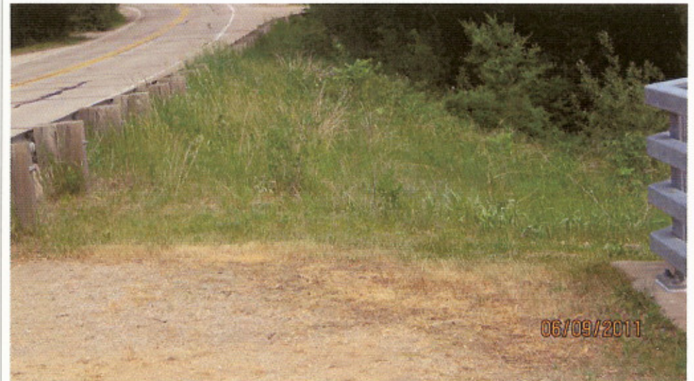
Left Side D/S Embankment (0009300609201108)
