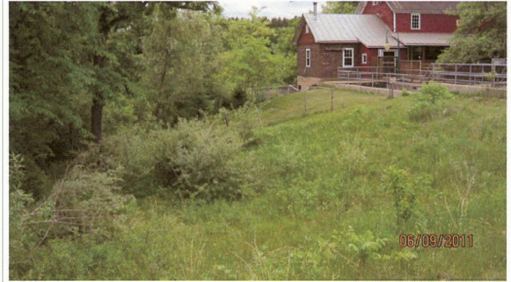
Left Side D/S Embankment / Powerhouse (0009300609201114)
