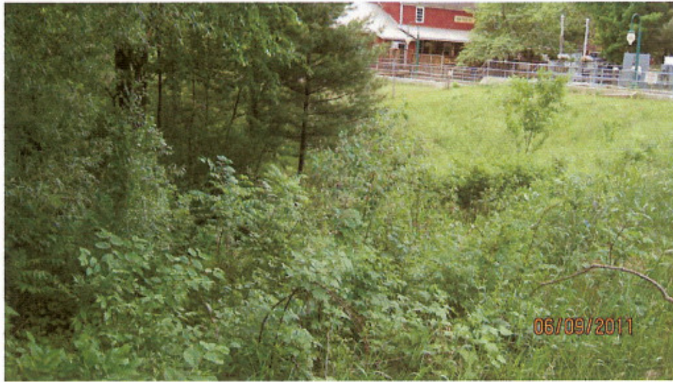
Left Side D/S Embankment (0009300609201113)
