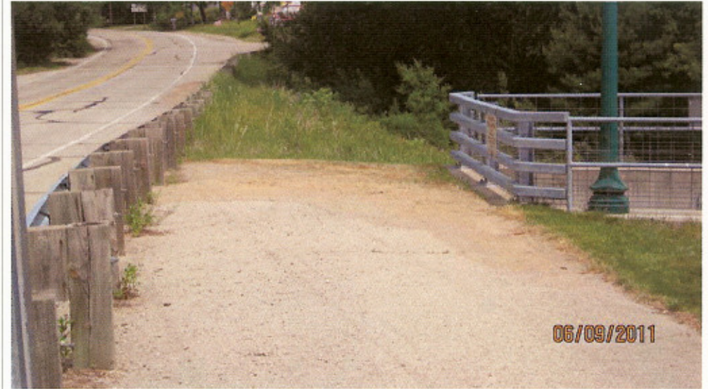
D/S Embankment / Flume (0009300609201106)
