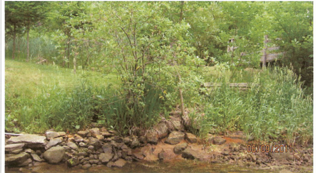
D/S Tailwater Channel Left Side (009300609201133)
