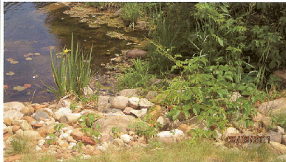
U/S Right Side Headwall Rip Rap (0009300609201104)
