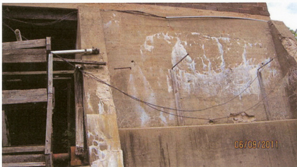
Rear Powerhouse Foundation Wall (0009300609201129)
