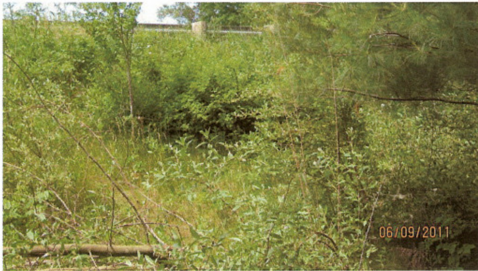
Left Side D/S Embankment - North (0009300609201109)
