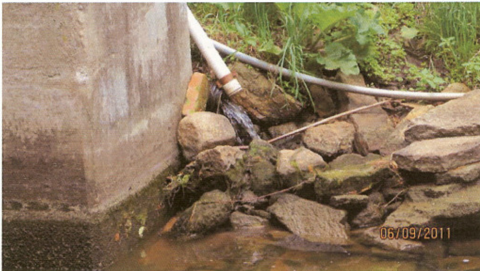
D/S Left Side Toe Drain (0009300609201121)
