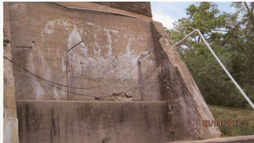
Rear Powerhouse Foundation Wall (0009300609201128)
