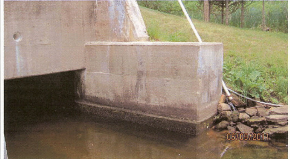
D/S Left Abutment (0009300609201124)
