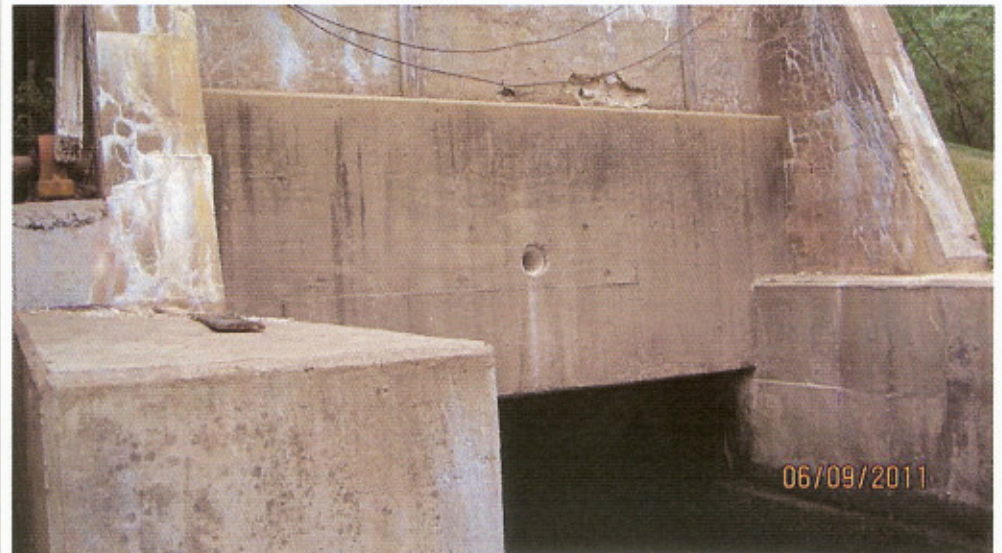
Rear Powerhouse Foundation (0009300609201126)
