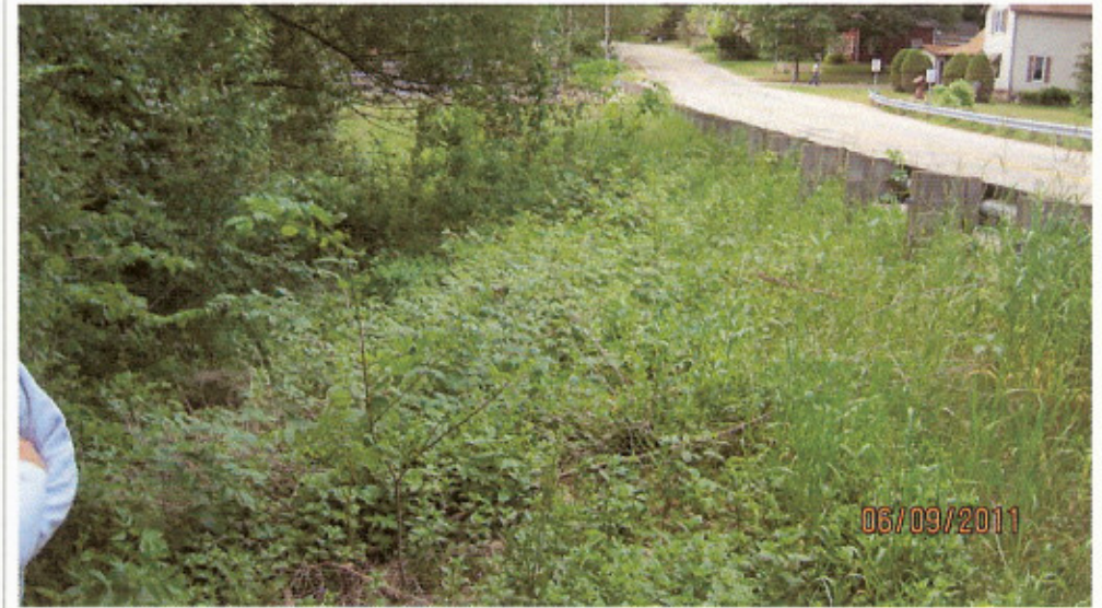
Left side D/S Embankment - Southwest (0009300609201110)
