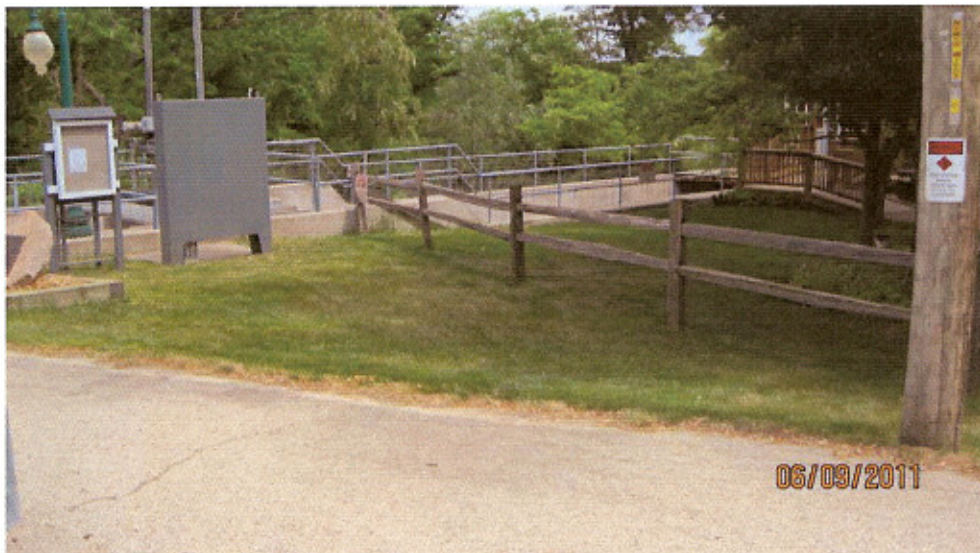
Right Side D/S Embankment (0009300609201159)
