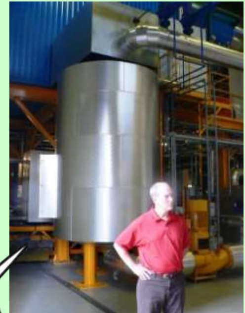
20 MW electric boiler
